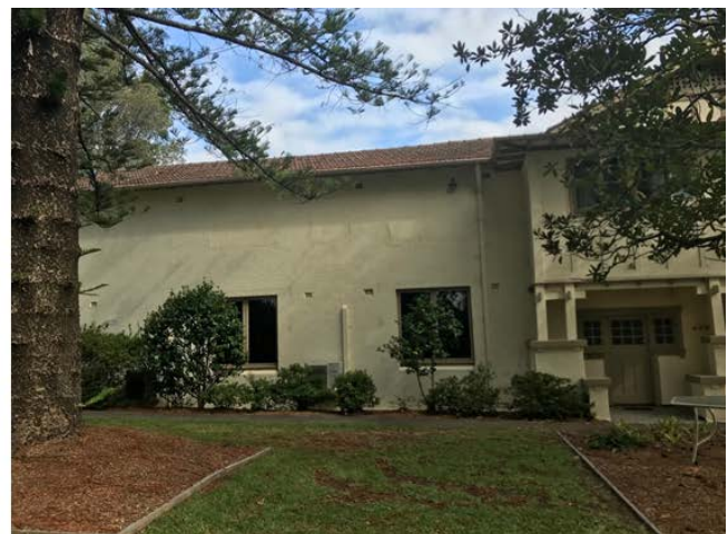
Photograph of Headfort House taken March 2018. Infilled windows apparent on the first floor.
