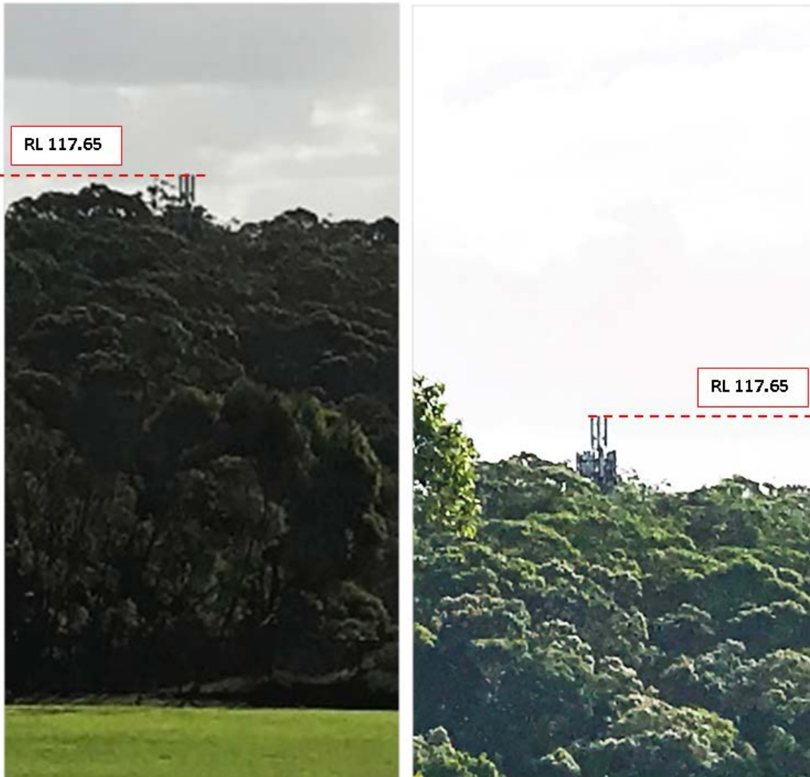
Optus Base Station at RL 117.65 visible above tree canopy. Photo taken from Lindfield Soldiers Memorial Park and oval. The proposal seeks an increased height to RL 127.3 making it highly visible above the canopy.
